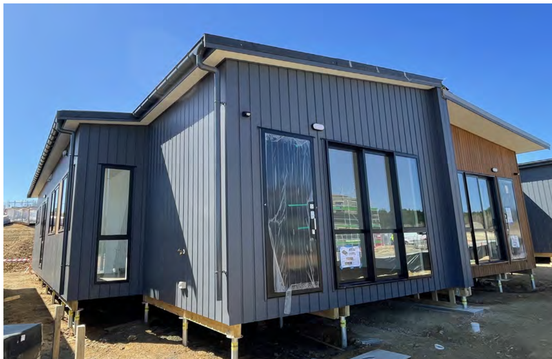
Figure 1.3: Ground below a piled foundation requires less earthworks than a concrete foundation.
