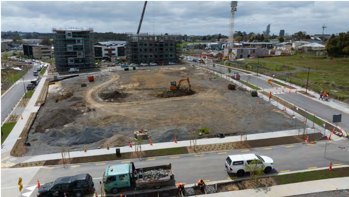
Figure 3.1: A Kāinga Ora housing development site in Northcote, Auckland. Topsoil is removed and the entire site is compacted to create 'good ground'.
