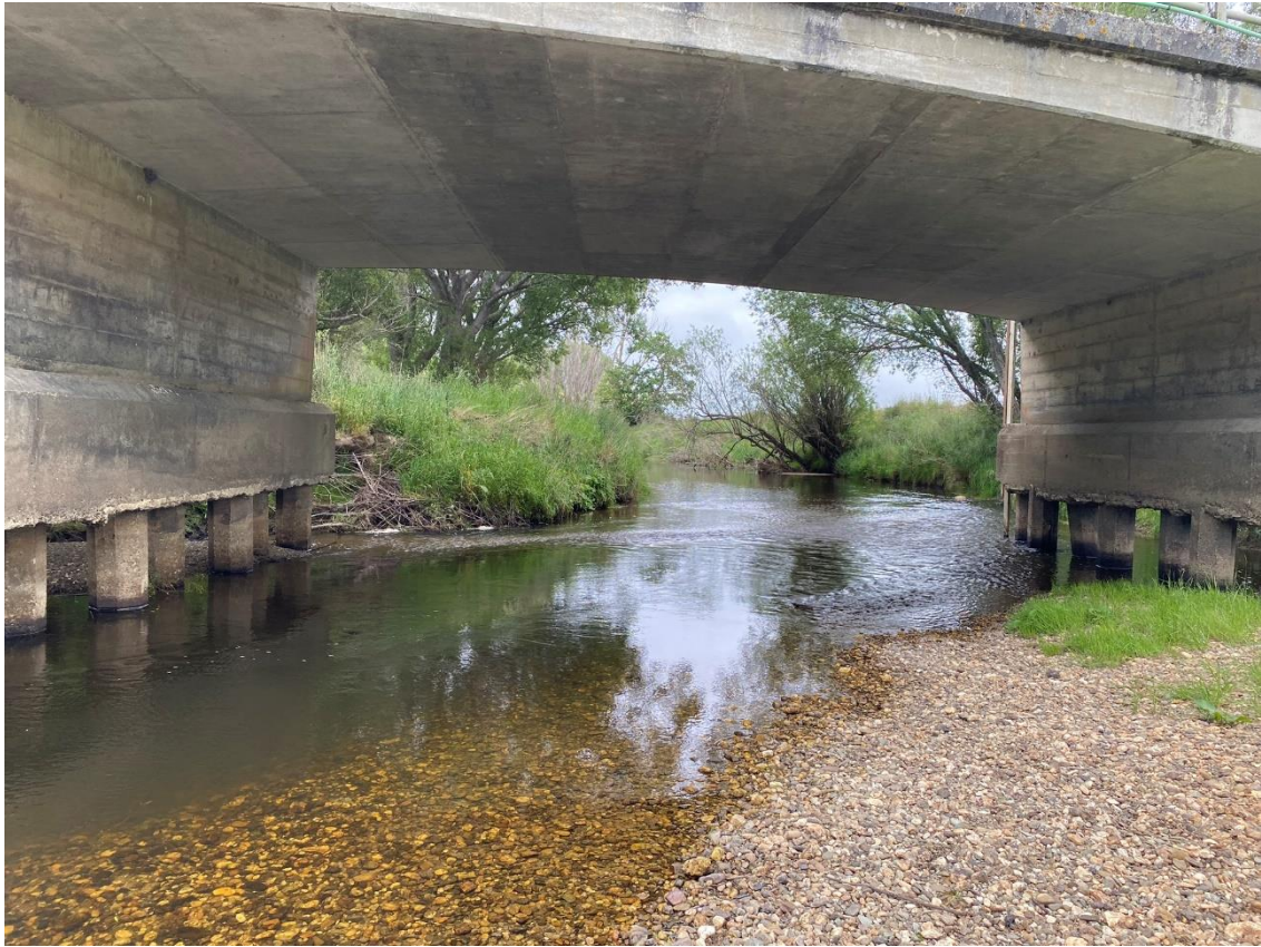
Figure 15: Downstream at the Waikāhahi site.
