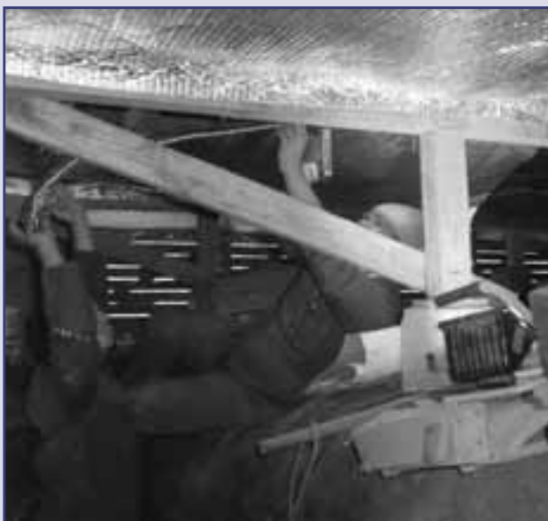
Underfloor insulation installation in the Waihi community
