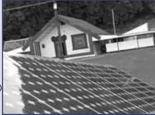
Solar panels at Tapeka Marae, Waihi
