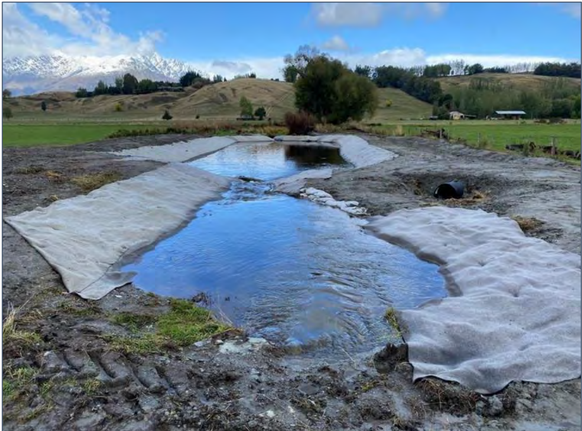
Figure 29: Sediment trap constructed by Mana Tāhuna in the Te Wai Whakaata catchment, below the korowai of Pa ha raki known to many as Coronet Peak. (Source: Mana Tāhuna, 2023).
